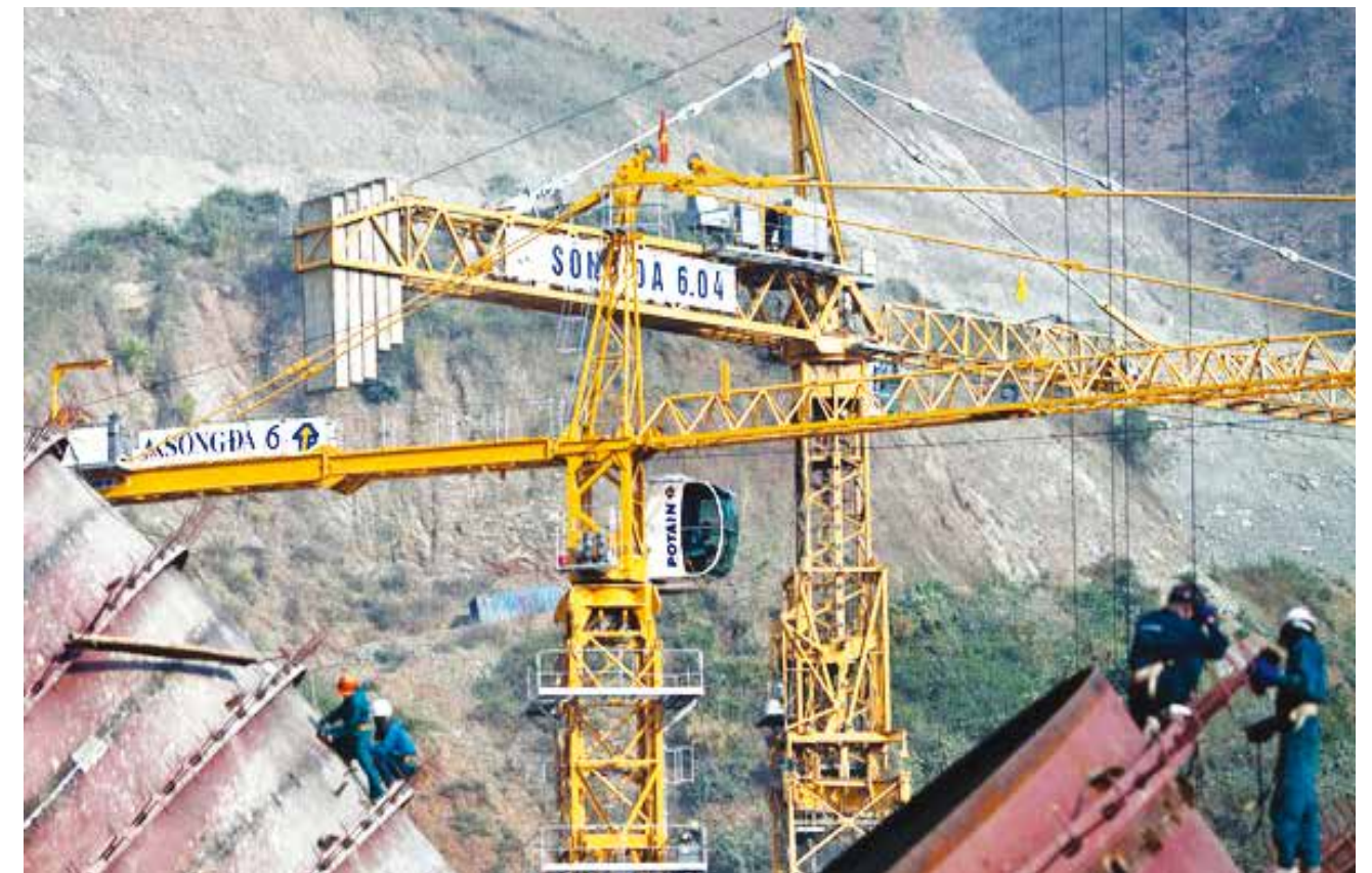
Potain Tower Crane at Se San 4 Hydropower Project
