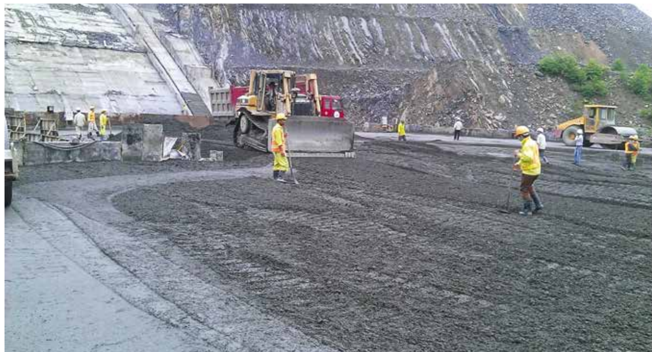
Roller Compacted Concrete work at Dong Nai 5 Hydropower Project
